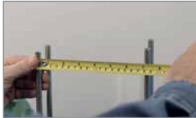
2. Measure the distance between the two V-brackets
